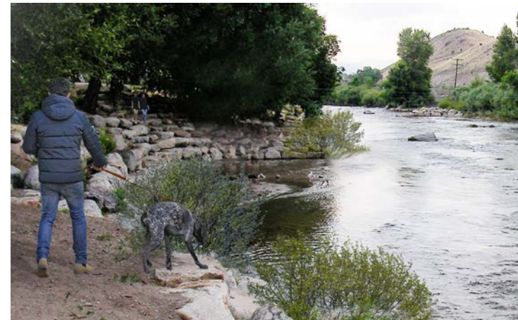
Type 2 Creek Access Point: Key creek access points located on existing, eroded cut banks along the trail network will be partially hardened and stabilized with rocks and deep rooted plants to facilitate access to easily eroded areas while protecting the creek.
